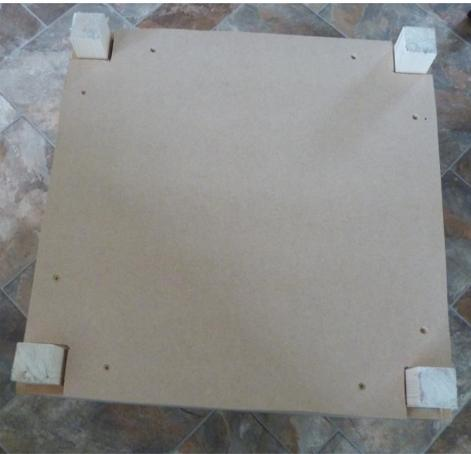
Use 9mm ply or MDF board for the base. This is 43 x 43 cm with 4 cut-outs for the legs as shown below. This is held in place by 8 screws, 2 screws each into the four horizontal struts at the base.
